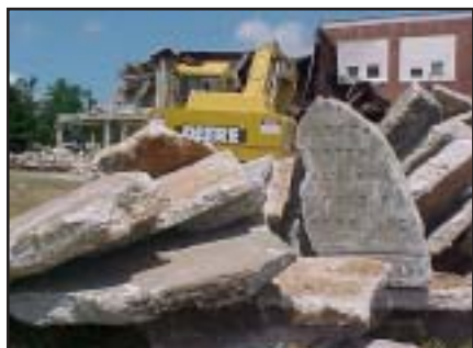
North Heights High School demolition.
